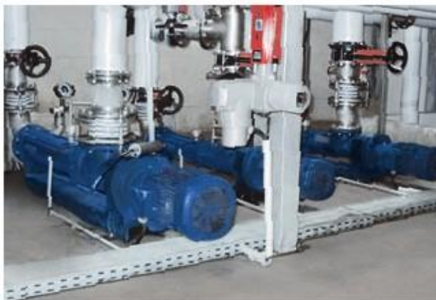
Pompe din seria BN 35-12 si BN 26-6L Produs vehiculat: Amestec de dejectii lichide si grasime Debit: 10–18 m 3 /h (44–79 GPM) • Presiune: 3–5 bar (43–72 PSI) Temperatura: 45–70 °C (113–158 °F)
